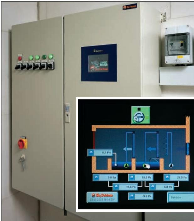
The electronic control system is responsible for the operational reliability and working safety of the whole facility. On the visual graphic screen all operational data can be displayed and controlled.
