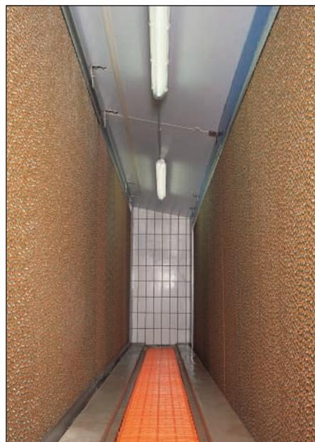
have to be closed during operation of the filter. A filter bank inspection aisle lies between filter banks 1 and 2.
