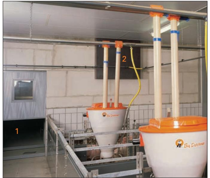
Air enters via door ventilation (1) and is directed into the central main drain via exhaust air valves (2)
