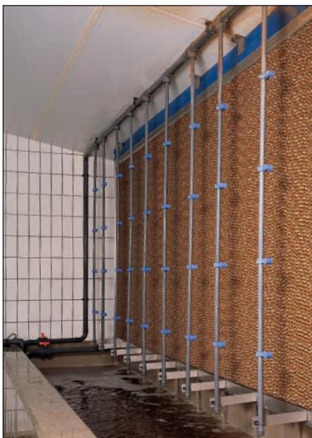
Nozzle groups spray water onto the front of the filter bank so that dust cannot cling to the filter bank. The individual filter chamber doors
